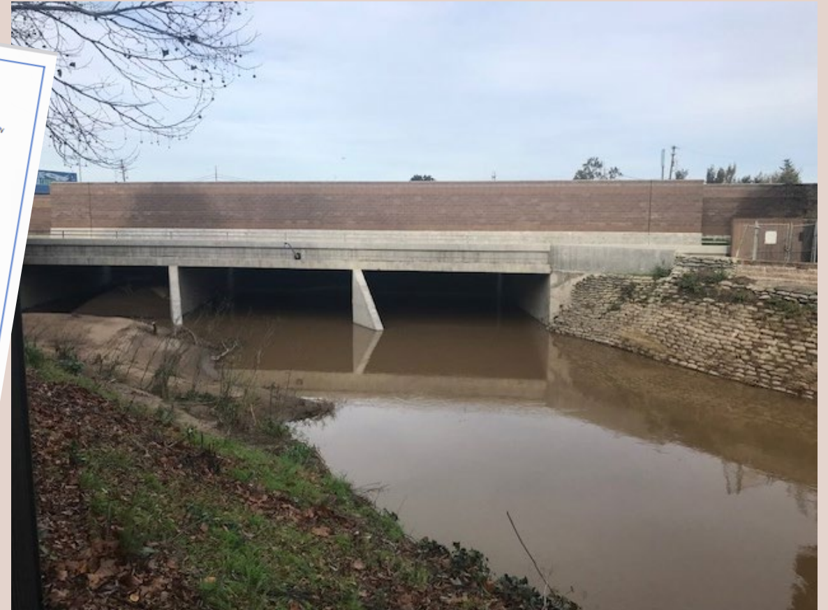
Hwy 101 Bridge over San Francisquito Creek
