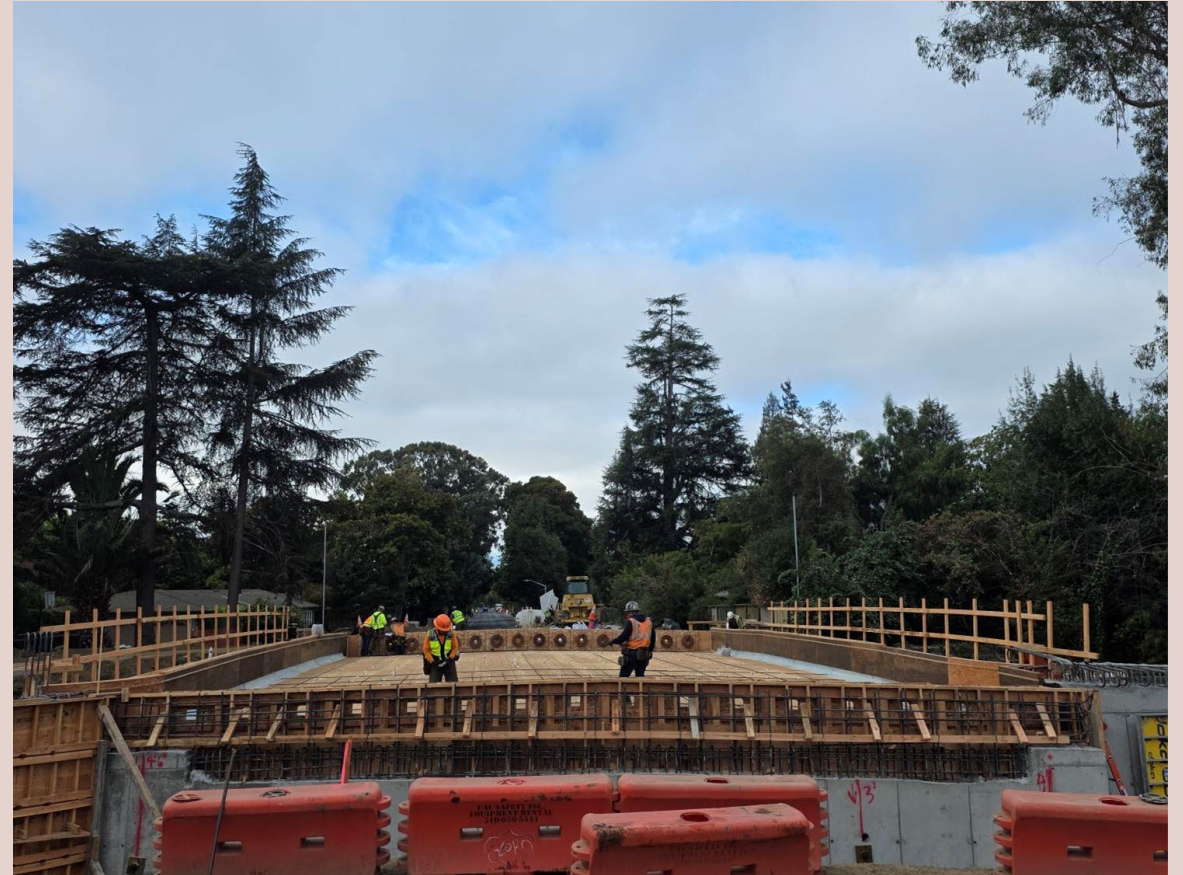
New bridge deck
