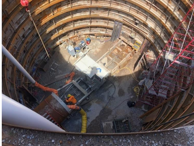
Figure 4-3 Typical Microtunnel Launch Shaft
