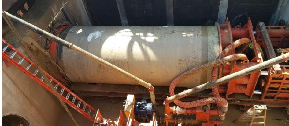
Figure 4-5 Typical Microtunnel Excavation and Pipe Jacking Operations
