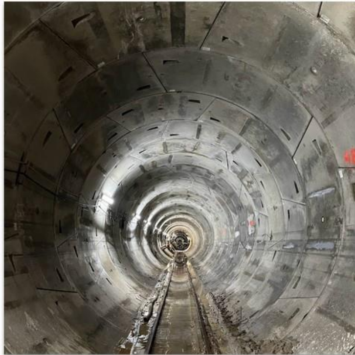
Figure 4-2 16ft diameter PCTL installed at the 3RPORT Combined Sewer Overflow (CSO) Tunnel project in Fort Wayne, IN.
