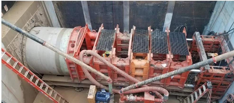
Figure 4-6 Typical Microtunnel Pipe Installation
